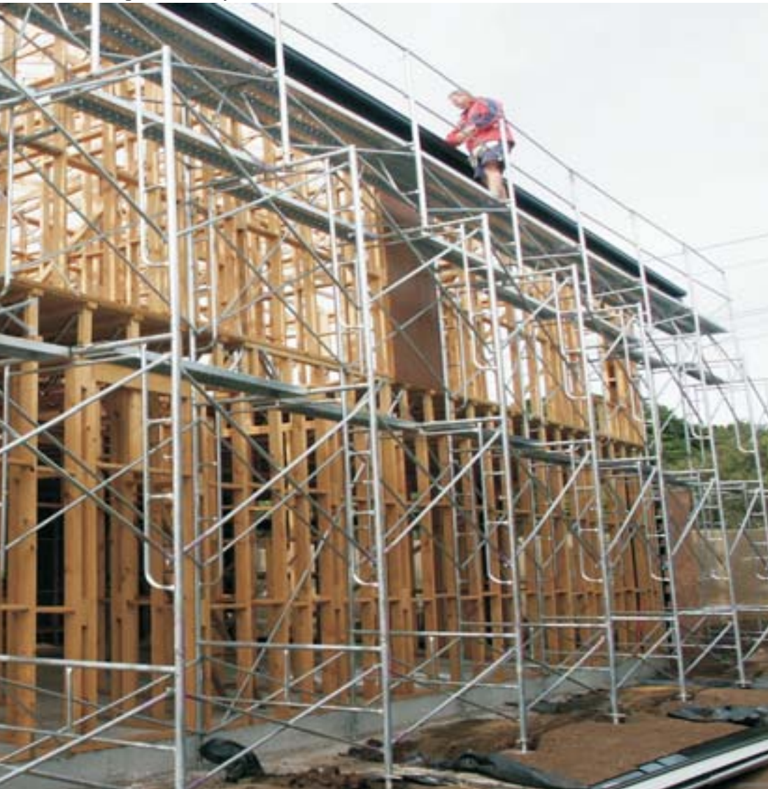
No tools needed to erect Modular Frame Scaffold
