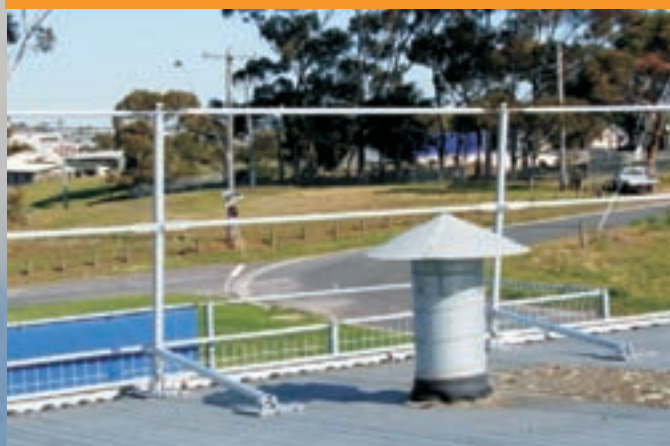
Roof Guard Rail
