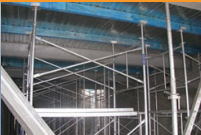
Shoring Jacks / Formwork
